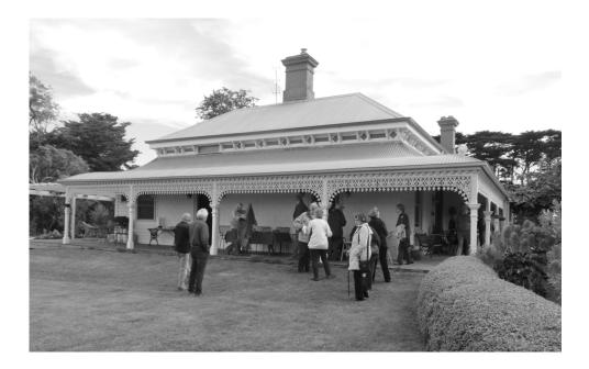
The original iron lace work that had been found in a shed has been successfully sandblasted clean, painted and then placed on the veranda. It makes a lovely addition to the corrugated iron roof.
