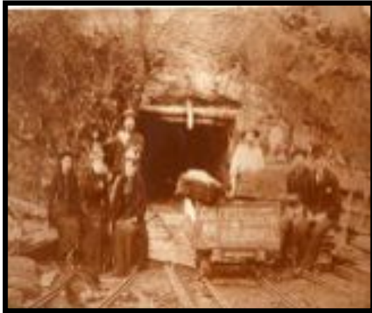
Coal Creek Proprietary Co. Mine
