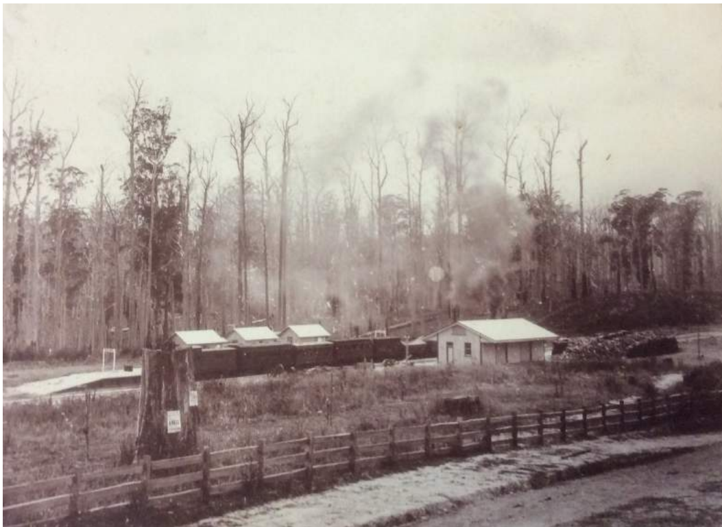
Bena railway station
